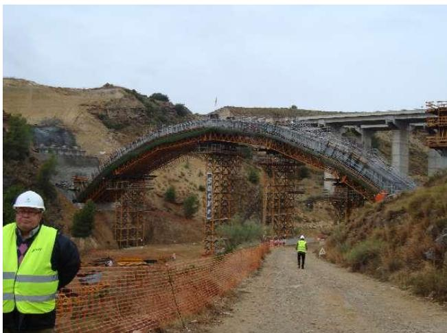
Back on the coach, we travelled a few miles to the part constructed bridge over the river Jauto. This is an interesting project. A semi-circular supporting arch has been built and the actual bridge will be supported by the arch.
